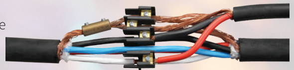
16mm 2 single core neutral screen to 16mm 2 4 core XLPE
